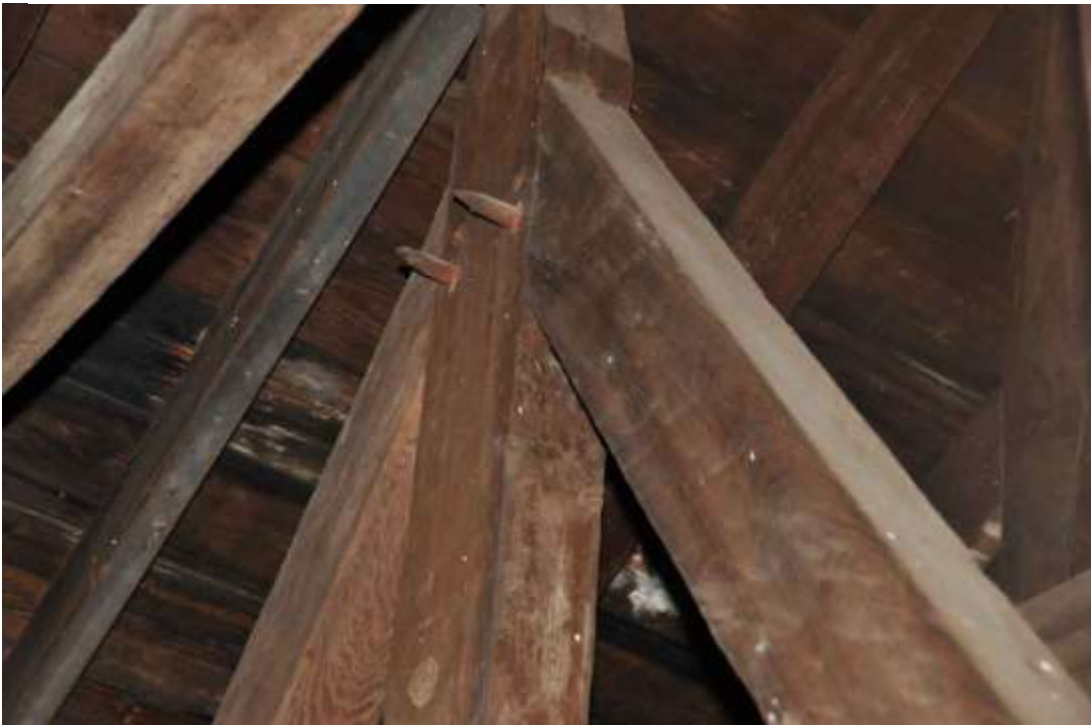
Norman Truss Construction in the Attic
