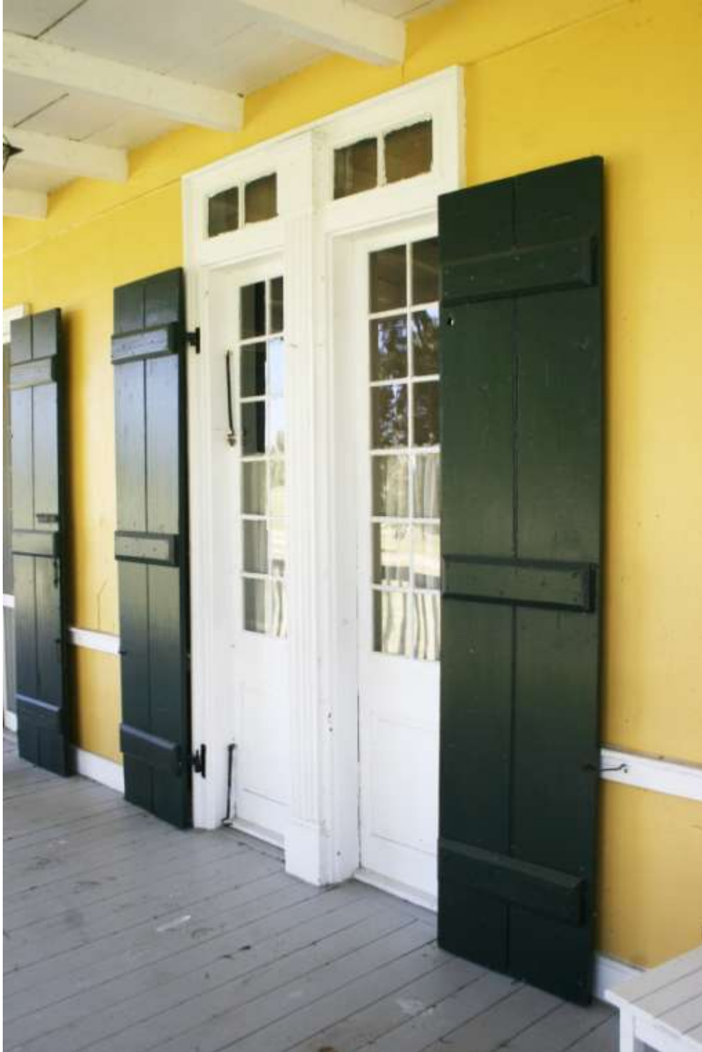
Unusual Federal Creole Second Floor Main Entrance
